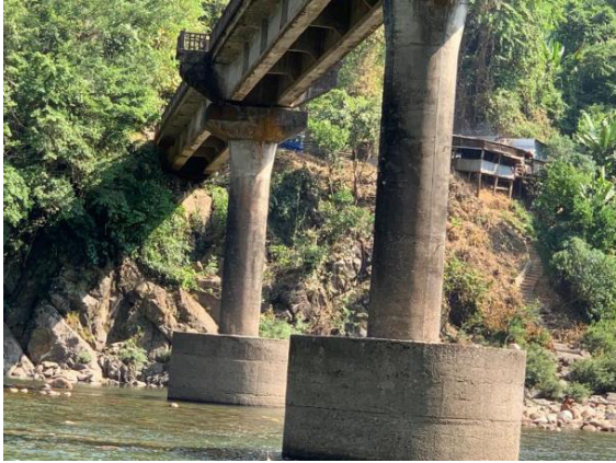
Figure 2: Pier heights are 8.4 meter each
