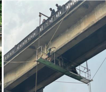
Figure 5: Suspended platform for physical access and NDT at site
