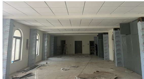
Fig.9 – Finished after strengthening
