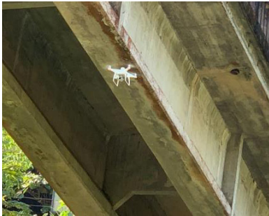
Figure 3: Drone Survey at the site for RVS with remote access
