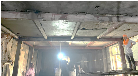
Fig.8 – Structural Steel frame
