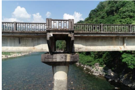
Figure 4: Drone accessing difficult locations for RVS - Pier Top
